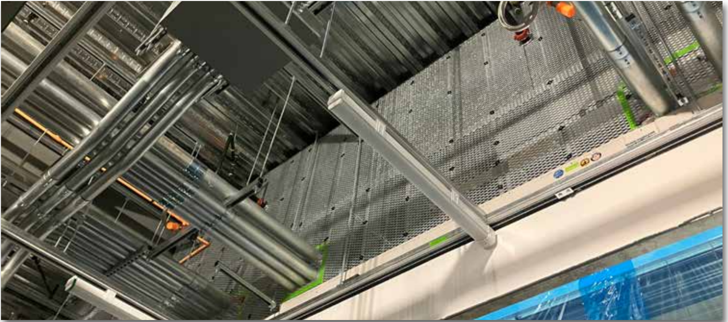
ASM .75-9F HM Super Max Security in optional hot dipped galvanized finish installed at Data Center
